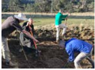
Digging foundation for water tank
